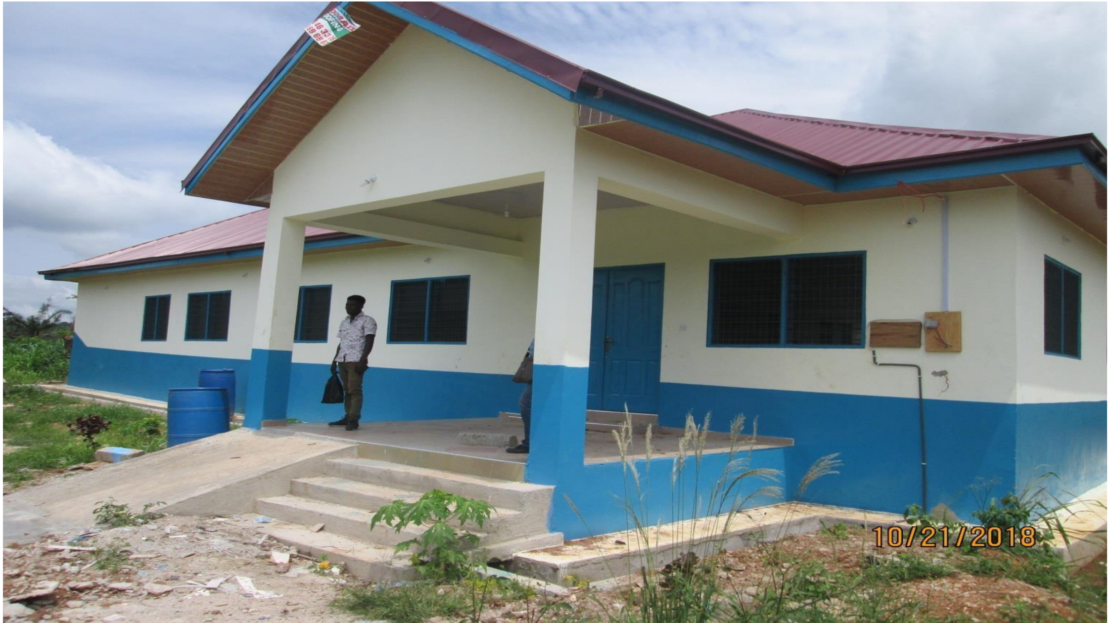
MATERNITY CENTER WITH MECHANIZED BOREHOLE AT FAWOMAN, AHAFO ANO SOUTH DISTRICT
