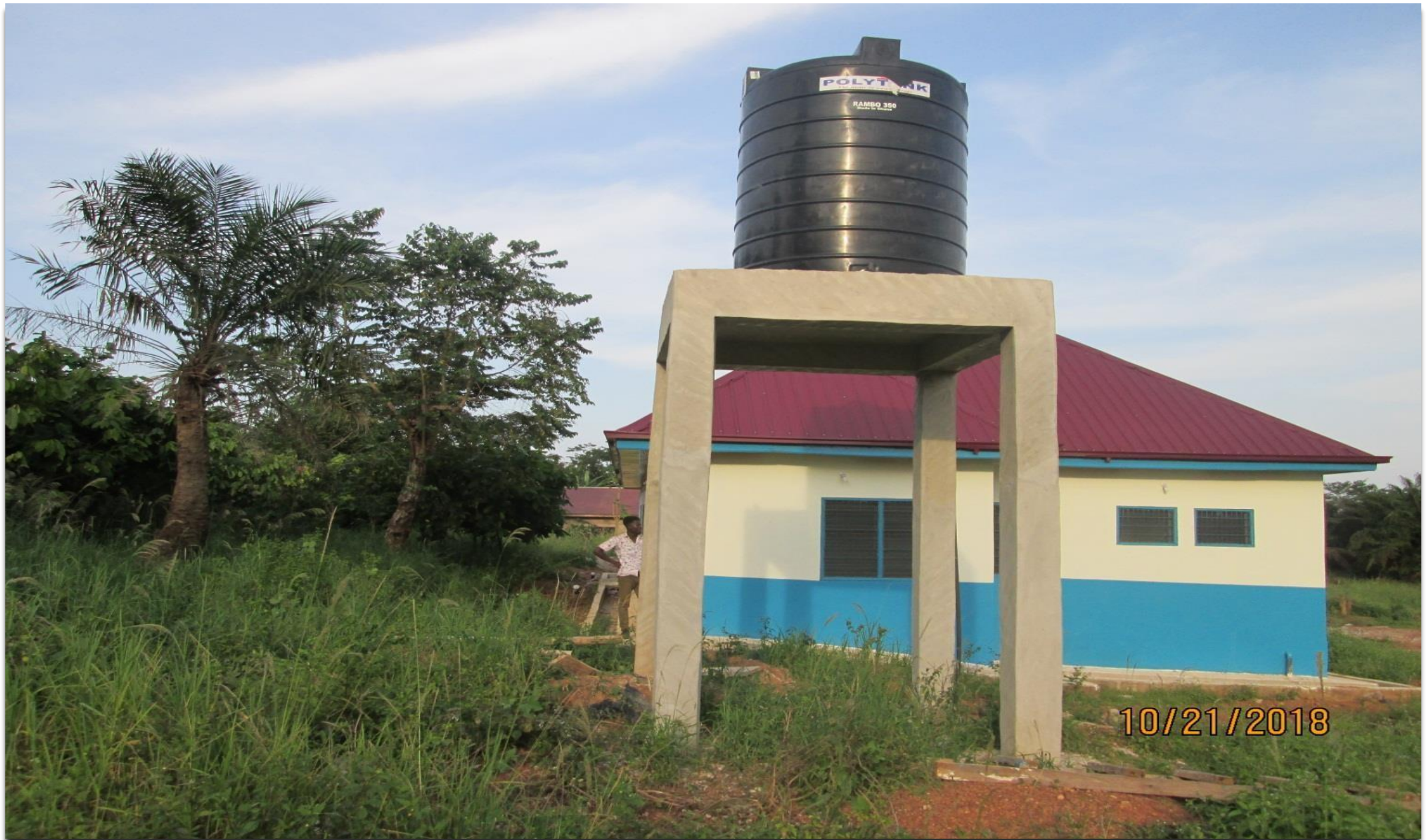
MECHANIZED BOREHOLE ATTACHED TO THE RURAL CLINIC AT KUNSU CAMP, AHAFO ANO SOUTH DISTRICT
