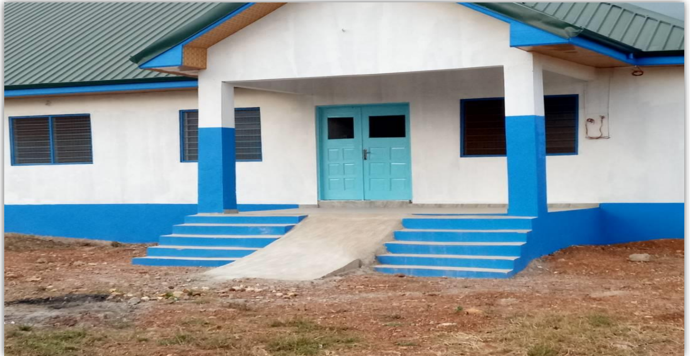
MATERNITY HOME WITH MECHANIZED BOREHOLE AT ABUTIA KISSIFLUI, HO WEST DISTRICT
