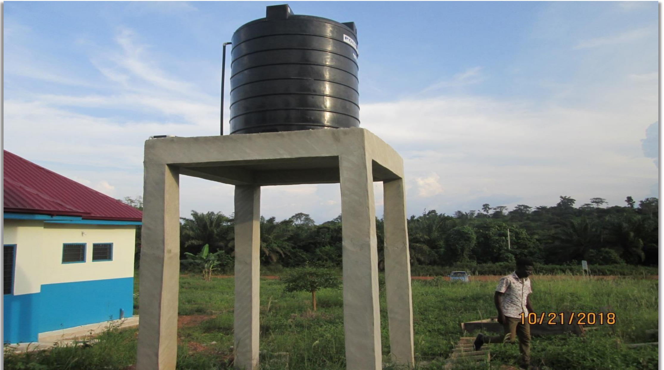
MECHANIZED BOREHOLE ATTACHED TO THE RURAL CLINIC AT WUROMSO, AHAFO ANO SOUTH DISTRICT
